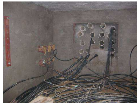
Waterproofing of air ducts inside the Olympic Sport Arena with KÖSTER products.
