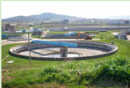
Sewage treatment plant, Istanbul, Turkey
