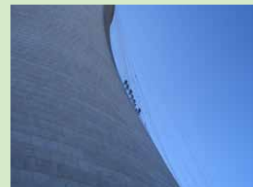
Cooling towers of a power plant, China
