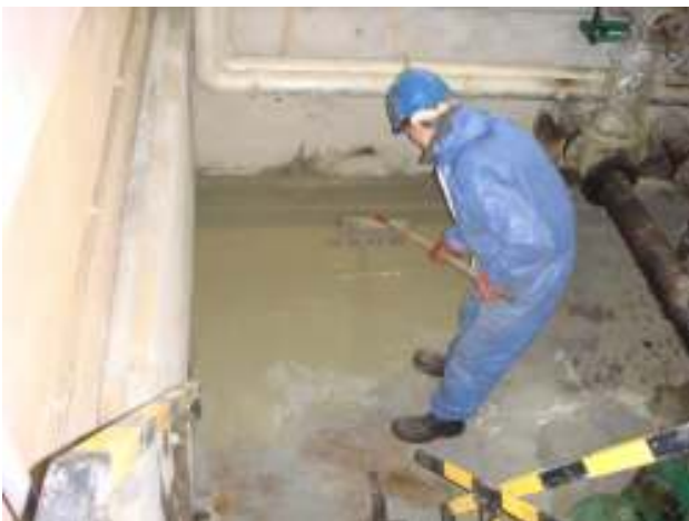
Gints is using the spinney roller (also a Koster product) to remove all trapped air and bubbles in the underlayment.
