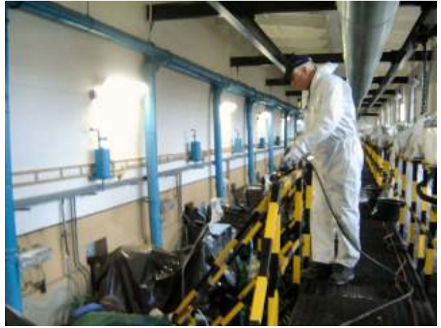
Aleksandrs supervises from the catwalk and manages the high pressure hose for Gints below.
