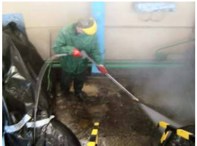
Due to the restricted space in these areas, the crew was unable to use a floor spinner, so Gints is using a high pressure water wand to clean and remove oil. Note face protection.
