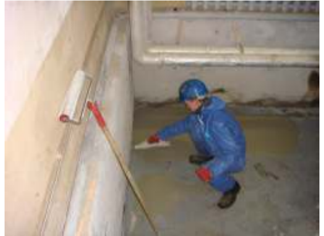
Gints trowels the underlayment into the corner. Note spinney roller leaning against the wall.
